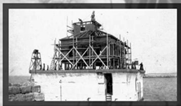
Construction of Superstructure-1934
